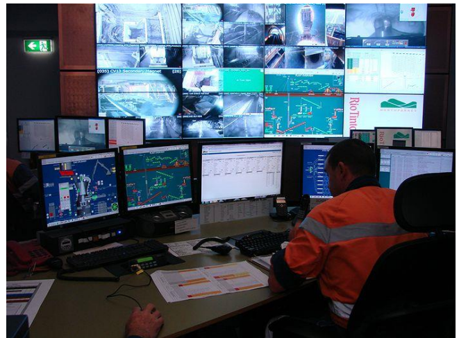
Figure 2 - North Parkes Mine (Australia) Control Room
