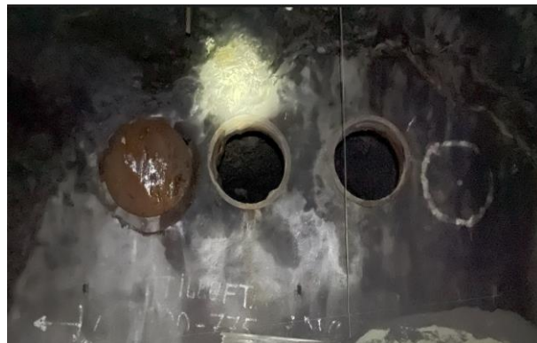
Type of blockage between the old shafts and its connection
